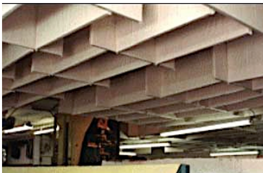
Figure 3: Installed sound absorption paneling. Image courtesy of U.S. Department of Labor Image Library .
